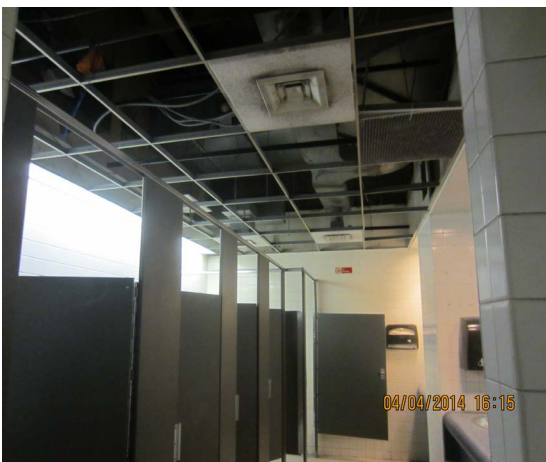
2nd floor rest room preparing for duct demolition
