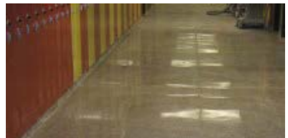
Concrete floor finish proposed by SBLM architects for Art & Music sculpture studio
