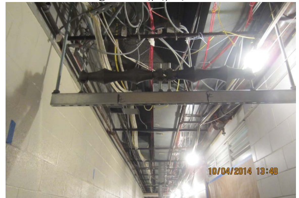
Install, rod, hangers and rollers for chiller pipes install
