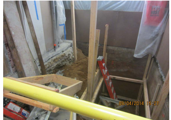
Excavation in pit -basement level
