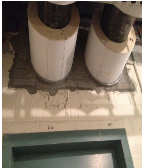
Firestop @ openings through walls.
